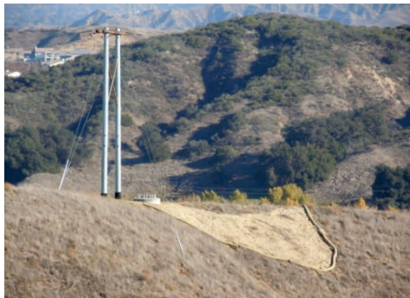
Figure 22 — Newly installed fiber rolls at a foundation site.
