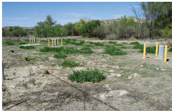
Figure 29 — View of the HDD restoration area. March 12, 2014.
