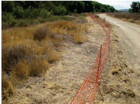
Figure 2 — Exclusion fencing placed around smooth tarplant populations adjacent to planned culvert installation on the El Casco Substation access Route. The photograph faces east toward the substation site.
